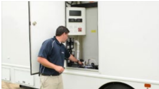
Pressure Gauge in Unit.
