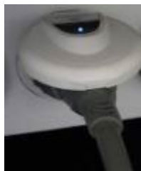
Check Blue Light on Trailer
