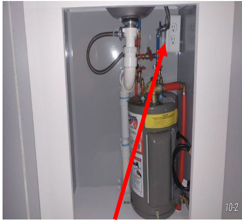
Plug in Water Heater
