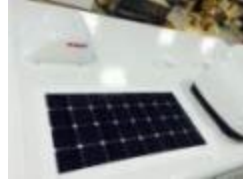
Solar Panel (Roof)
