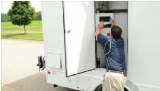
Removing Fuse Panel
