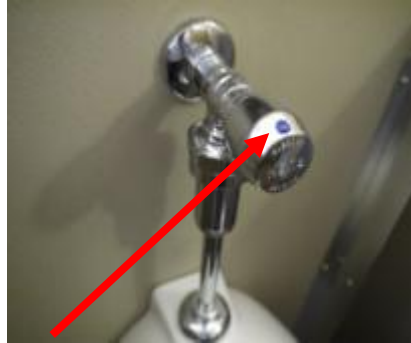
2. Remove Cap and Screw
