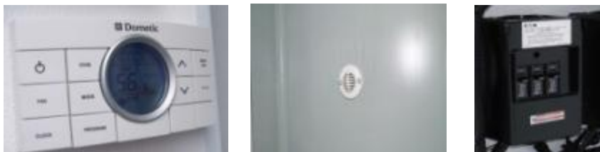
1. AC/Heat Control Panel 2. Thermostat Sensor 3. AC Breaker
